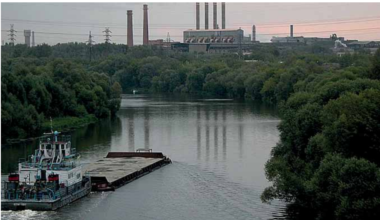
Lafarge Voskresensk Cement Plant
